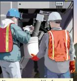
New processes like foamed or expanded as phalt base stabilization require ongoing testing during construction; here half-life of asphalt foam is tested by extraction into bucket and how long it takes to reduce by half
