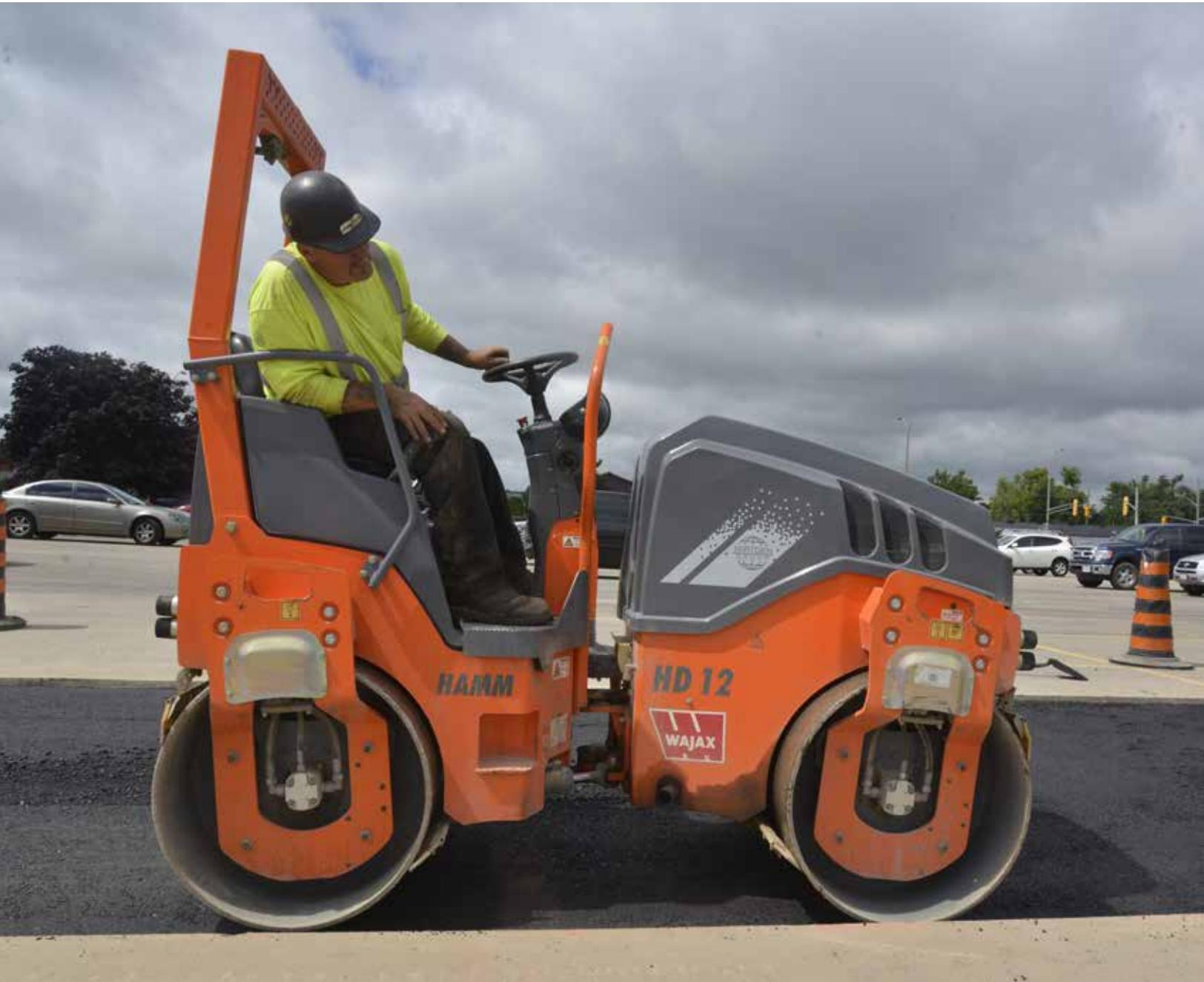
The vibrating screed was getting about 90 percent compaction ahead of finish rolling by a Hamm HD 12 CompactLine roller.
