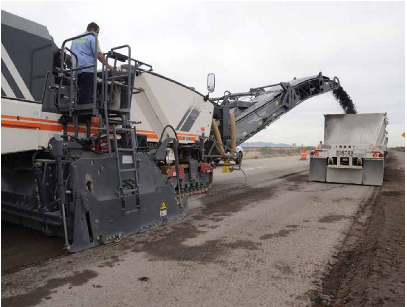
LEFT: "The grade control has seven points of control, and what we really like is that it's holding the 2 percent crossfall really well," Jason Torres said. RIGHT: "When we are dumping on the shoulders, were getting a 25 percent improvement..." — Jason Torrese. BELOW: Las Vegas Paving uses the W 250i full-lane cold mill from Wirtgen to mill 27 miles in both directions on I-15 north of Las Vegas. The machine is Wirtgen's biggest cold mill and generates a total of 991 horsepower with two engines engaged while meeting Tier 4 Interim emissions regulations.
