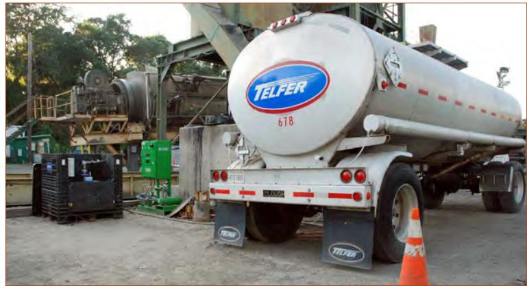
In central California, terminal blend of rubberized asphalt liquid is injected into production of warm mix asphalt
