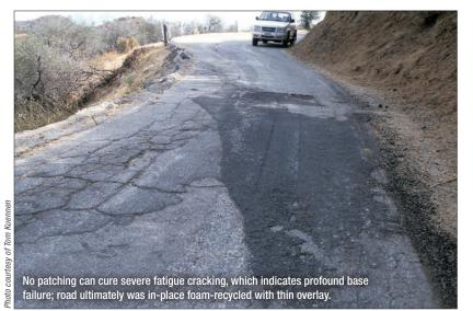
"[L]oad-related top-down fatigue cracking — i.e., cracking that initiates at the surface of the pavement and propagates downward — commonly occurs in hot mix asphalt (HMA) pavement," say Hong Joon Park and Y. Richard Kim, Ph.D., P.E., North Carolina State University-Raleigh, in their 2013 Transportation Research Board paper, Investigation into the Top-Down Cracking of Asphalt Pavements in North Carolina.
