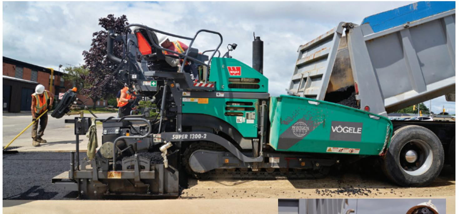
and biking paths, sidewalks, utility work and shoulder paving. Paving widths range from 2 feet 6 inches to 13 feet 9 inches, making the Super 1300-2 a very versatile machine.
