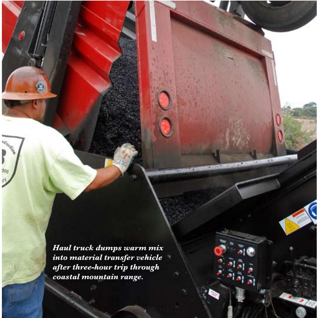
***Haul truck dumps warm mix into material transfer vehicle after three-hour trip through coastal mountain range.***
