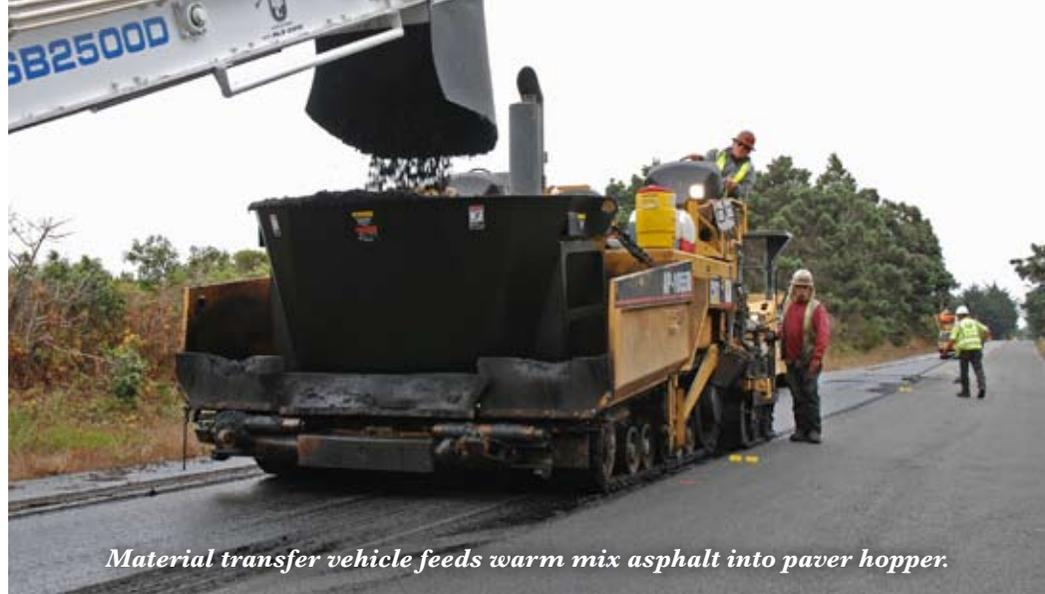
*Material transfer vehicle feeds warm mix asphalt into paver hopper.*
