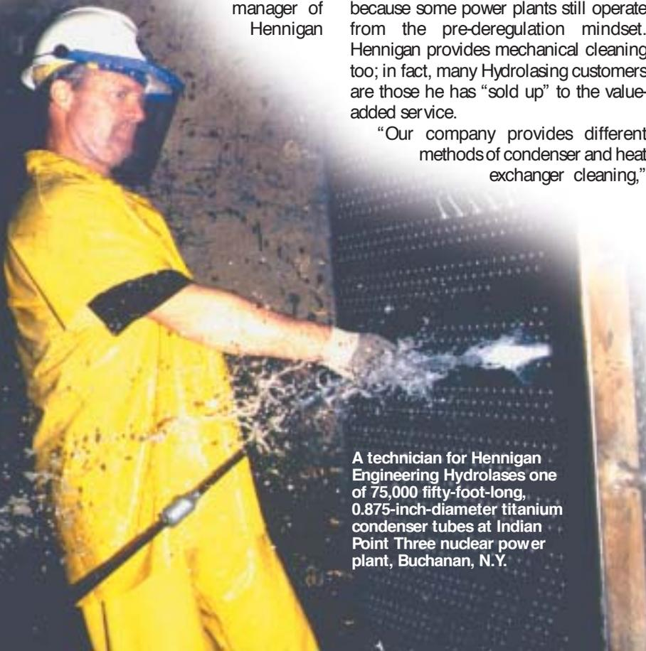
A technician for Hennigan Engineering Hydrolases one of 75,000 fifty-foot-long, 0.875-inch-diameter titanium condenser tubes at Indian Point Three nuclear power plant, Buchanan, N.Y.
