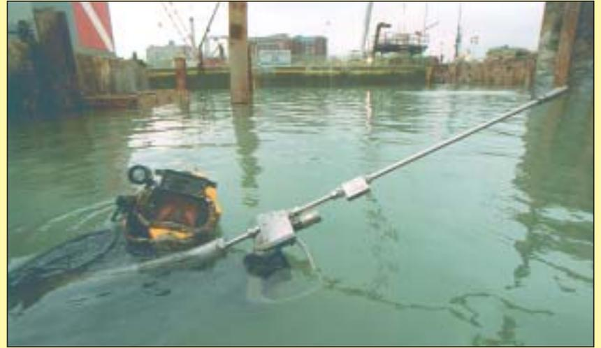
**A diver with Hennigan Engineering Hydrolasing equipment by Jetstream of Houston descends into Boston Harbor to remove concrete overpours on a tunnel foundation, as part of Boston's "Big Dig" Central Artery/Tunnel project. (Photo courtesy of Boston Globe)**
