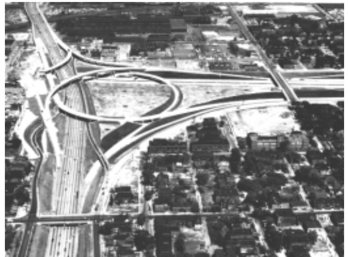
In Michigan, the interchange of I-75, the Walter Chrysler Freeway (right), with I-94, the Edsel Ford Freeway (top to bottom), nears completion in June 1964.
