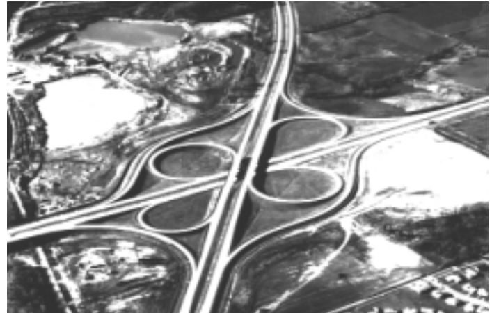
The interchange of I-74 and I-465 in Indiana nears completion in 1963.
