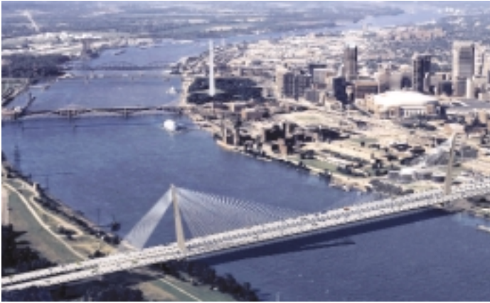
A rendering of the proposed new Mississippi River crossing on I-70 from Illinois (left) to Missouri at downtown St. Louis. The massive bridge project needs a funding compromise between the two state DOTs.
