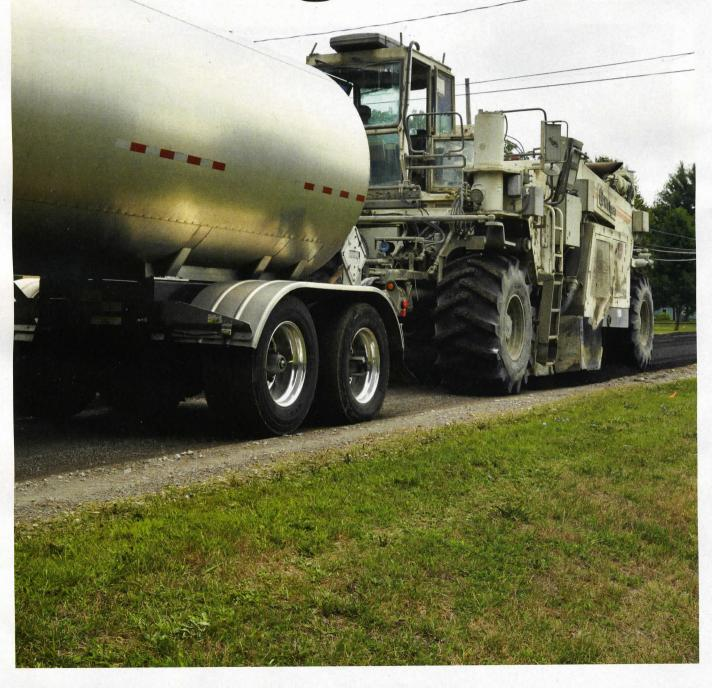
On the Monroe County, MI, full depth reclamation, engineered asphalt emulsion is injected into reclaimed materials as they are mixed.
