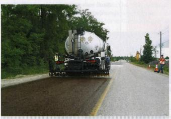
Surface treatments using asphalt emulsions can solve a variety of pavement problems that result from oxidation of oils in the binder and water penetration.
