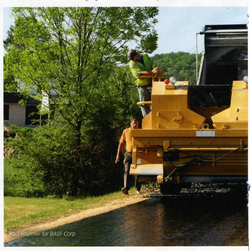
spraying a pavement surface with asphalt emulsion, covering this with a layer of stone, and repeating the process but using the same emulsion at a different application rate, and smaller stone. Compaction by rollers forces the smaller stone to interlock with the larger. Over the years this process has proven to be the best surface maintenance treatment for their roads, according to county engineer Corey Chambers.
