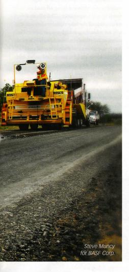
Forces of TxDOT District 15 place chip seal utilizing CHFRS-2P asphalt emulsion in May 2011.
