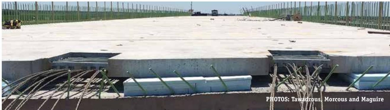
On precast bridge deck in Kearney, Neb., end panel showing post-tensioning anchorage block.
