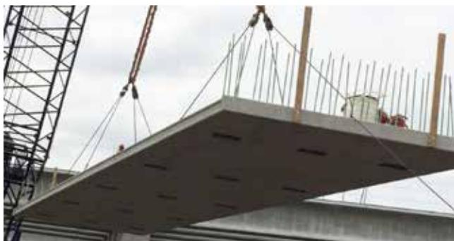
Panel lifting showing shear pockets on precast bridge deck section in Kearney, Neb.
