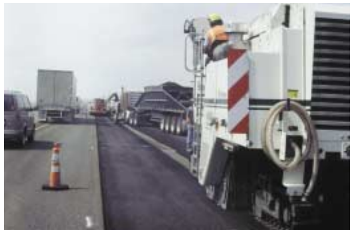
Milling preceded asphalt laydown
