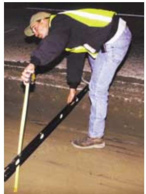
Douglas Asphalt's milling foreman Chris Thompson checks cut depth
