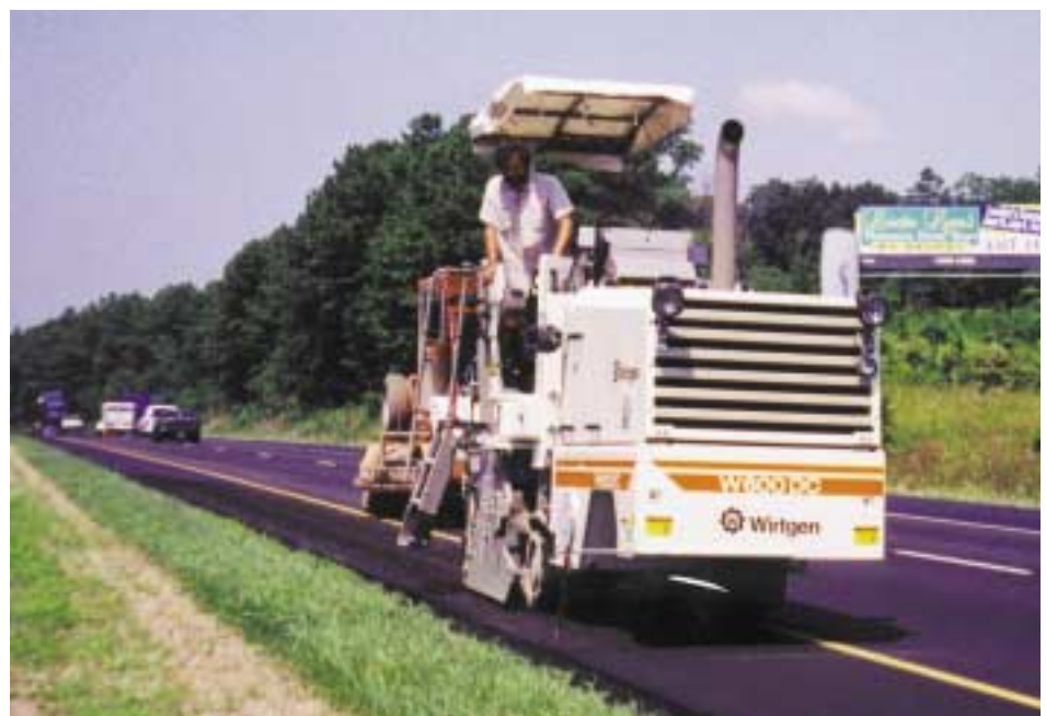
W 600 DC mills shoulder strips on interstate highway shoulder
