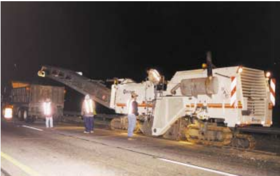
Heavy daytime traffic on I-475 necessitates night work
