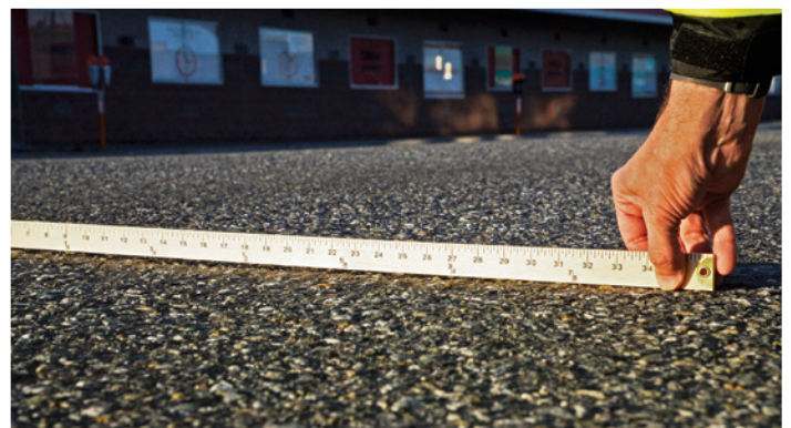
After four winter seasons (2015-2019), 200 block of E 5th Avenue with HiMA-modified PG 64-40 E binder shows minimal rutting
