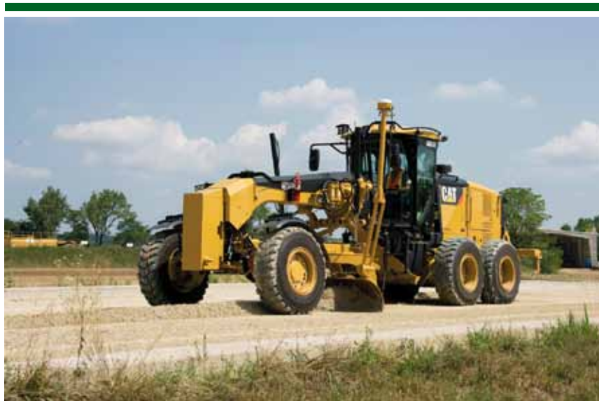
▲ New Cat 160M2 motor grader preps subbase prior to base placement.
