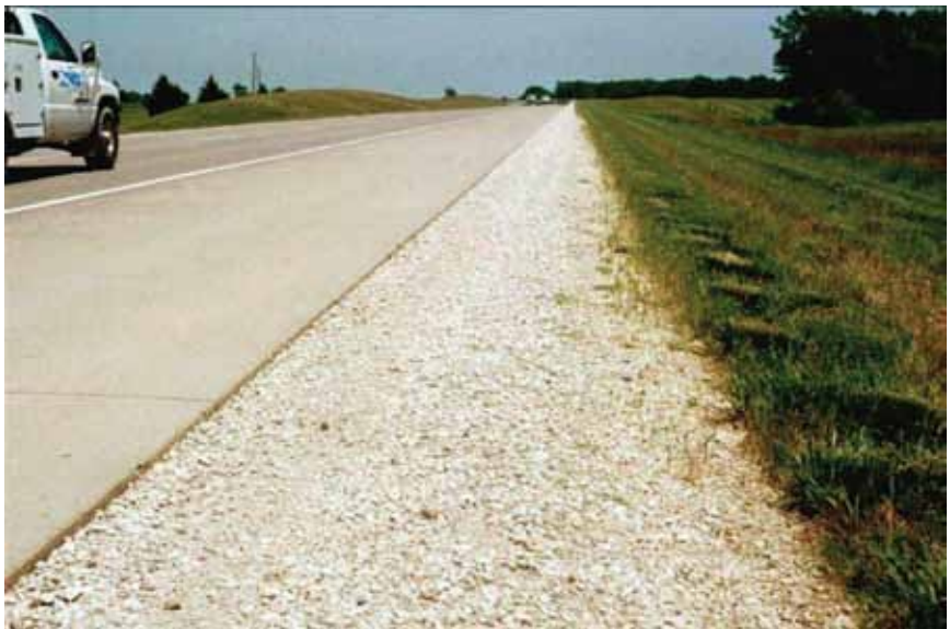
▲ "Daylighted" permeable base – exposed here at the shoulder – is a lower-cost PCC pavement drainable design that doesn't require separation fabric or drainage systems.
