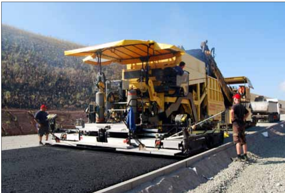
▲ Dynapac’s Compactasphalt system places two lifts of asphalt, hot-on-hot, using a single, large, modified paver and two compacting screeds
