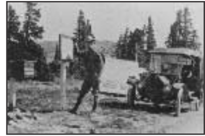
A.E. Palen, OPR senior engineer, on the job in 1918. Photo courtesy of FHWA.
