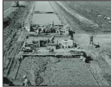
Concrete spreading process during the construction of Interstate 80 northeast of Seneca, Ill., in 1963. Photo courtesy of the National Archives.
