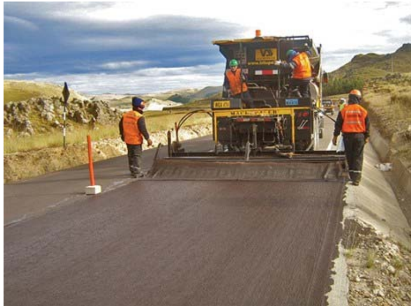
A VSS Macropaver Model 12B slurry machine in the Andes
