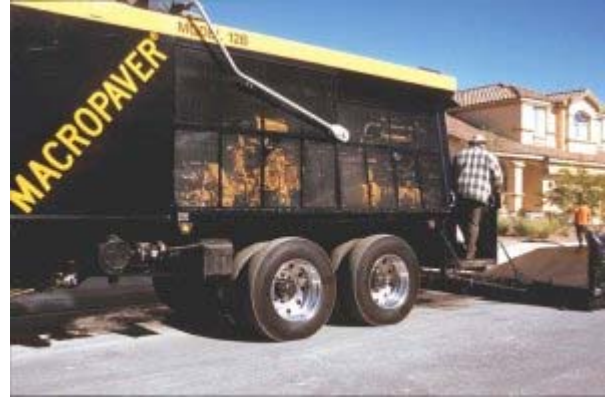
Slurry surfacings are popular pavement preservation treatment in American West and Southwest
