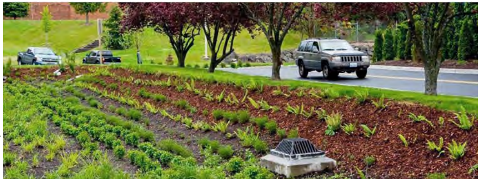
Drainage is an important element of sustainable design; here, in Tacoma, Wash., a roadside drainage swale keeps exhaust byproducts like residual hydrocarbon compounds and heavy metals from pavement surface out of water supplies. Natural bacteria in soil neutralize products in runoff prior to runoff reaching existing aquifer.
