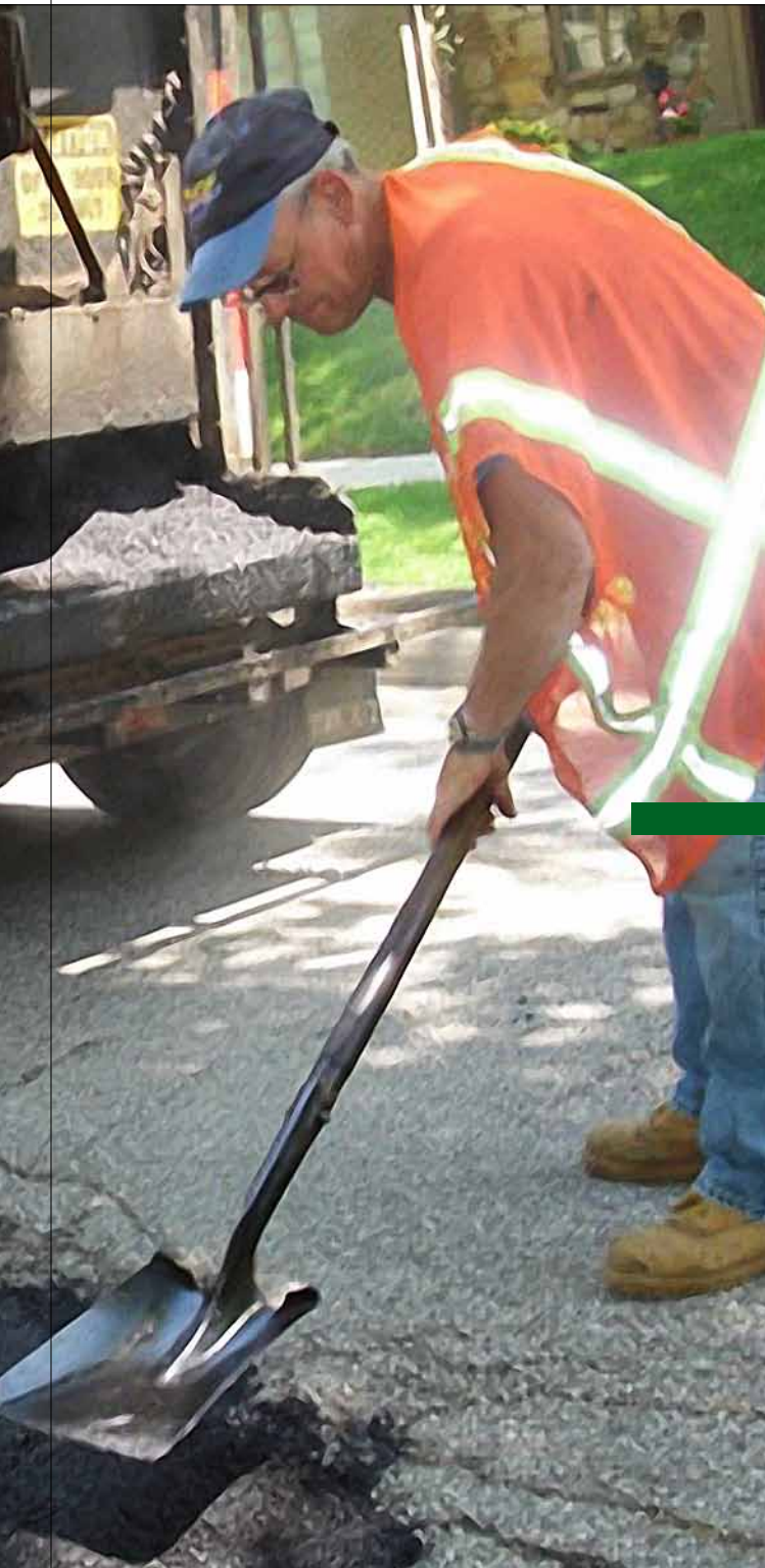
▲ Classic “throw, roll and go” patching is a time-honored, if hoary, solution to pothole repairs.
