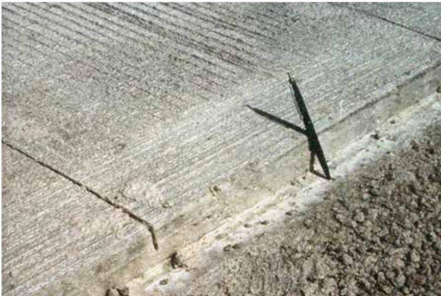
Section of very thin 2-inch textured concrete overlay on Iowa State Route 2.
