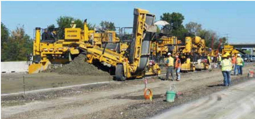
Illinois State Toll Highway Authority places test of two-lift, wet-on-wet concrete overlay on I-88 in 2012.
