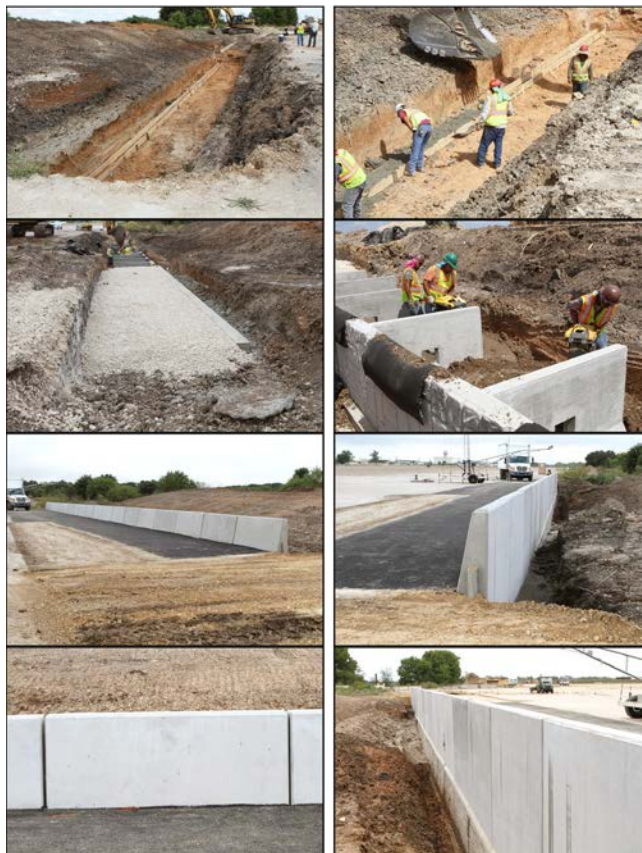
Installation of Gravix barrier prior to testing
