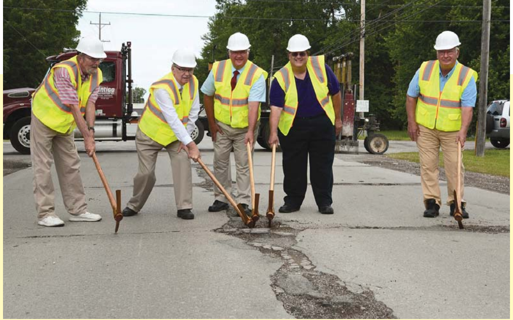
Right (top to bottom): (top) Members of the Monroe County Road Commission pose before evidence of the failed road during the project's groundbreaking; (middle) Initial breakup of the failed concrete panels; (bottom) The existing concrete was pulverized and an Iron Wolf crushed it in place.
