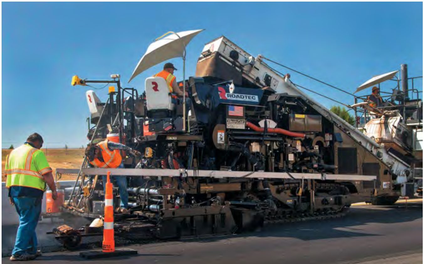
For ultrathin bonded overlay, asphalt emulsion bond coat from paver-mounted tank is placed on existing pavement directly in front of asphalt paver screed for hot-on-hot paving
