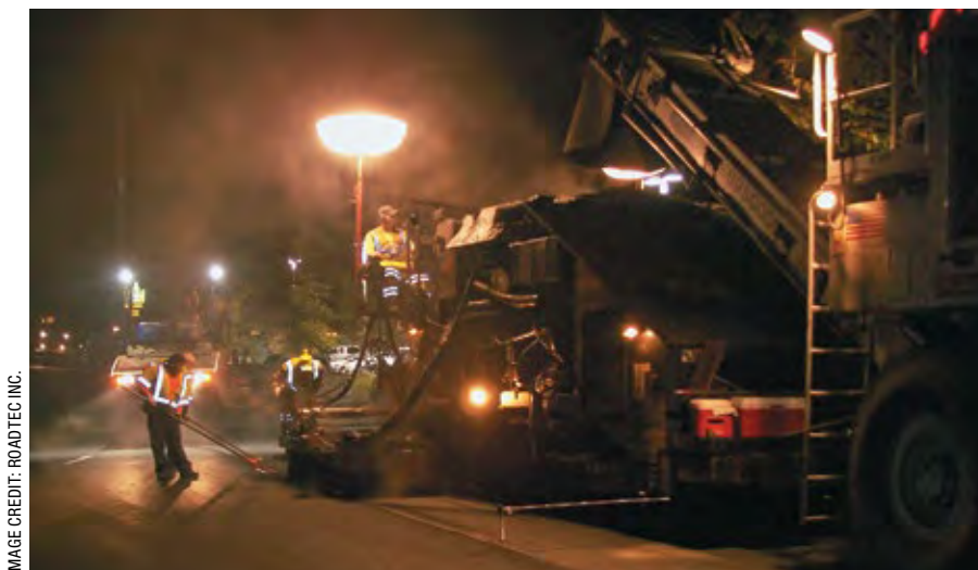
On Silverado Trail in Napa, Calif., asphalt emulsion bond coat is sprayed by Roadtec SP 200 spray paver immediately in advance of screed placing asphalt rubber modified UTBWC
