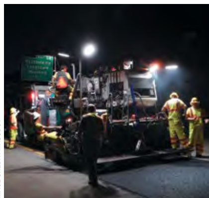
On mainline lanes of U.S. 3 in Massachusetts, spray paver places asphalt emulsion bond coat and ultrathin bonded overlay in one pass
