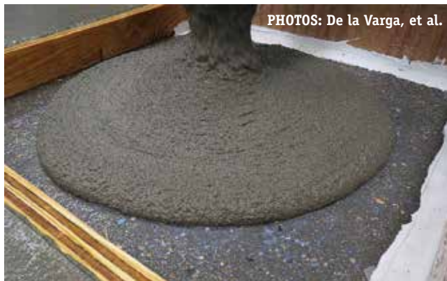
Following sandblasting of concrete slab, colloidal nanosilica suspension is applied by brush (left), followed by grout pour.
