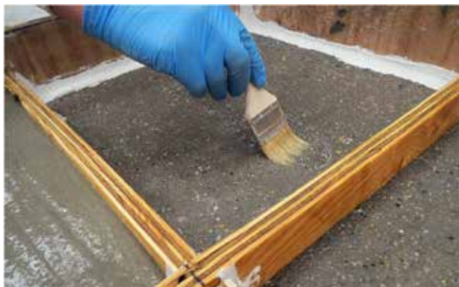
Following sandblasting of concrete slab, colloidal nanosilica suspension is applied by brush (left), followed by grout pour.
