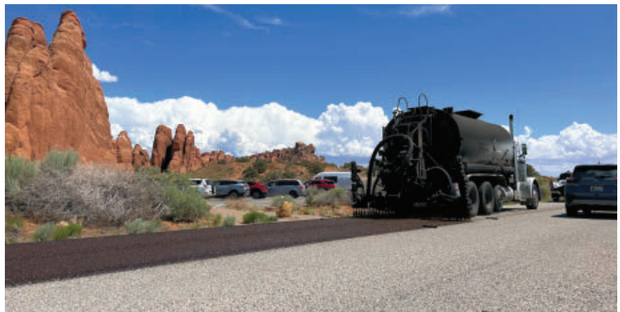
An emulsion fog seal goes over chip seal placed on national park road in Arches National Park
