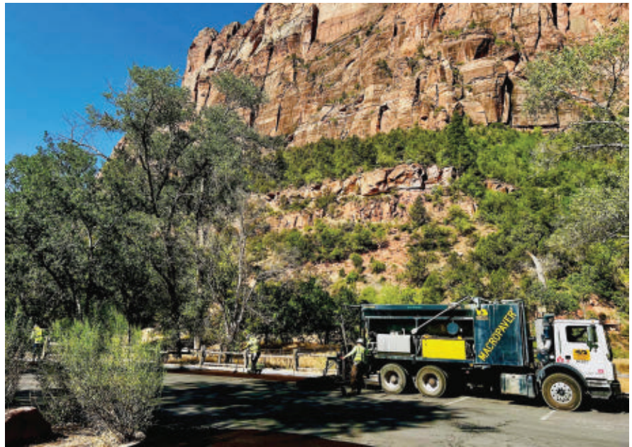
A Type 2 slurry seal overlay is placed at the day parking lot near the entrance of Zion National Park
