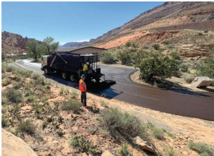
Crews place a Type 2 slurry seal overlay around a ranger station at Arches National Park
