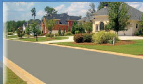
COOL PAVEMENT TECHNOLOGY
