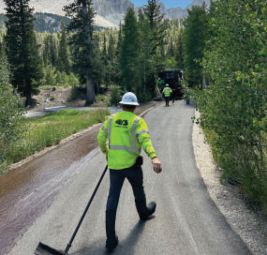
Type 2 slurry surfacing is placed at all campsites and campground roadways in Great Basin National Park
