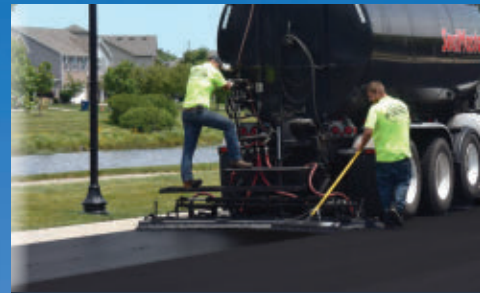
LIQUID ROAD SURFACE TREATMENT
