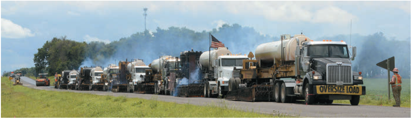
HIR process typically uses eight units, one after the other, slowly moving forward and gently heating the existing asphalt pavement to the optimum level
