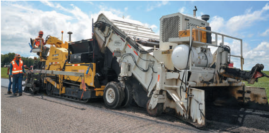
Windrow elevator places hot-recycled mix with rejuvenator into paver
