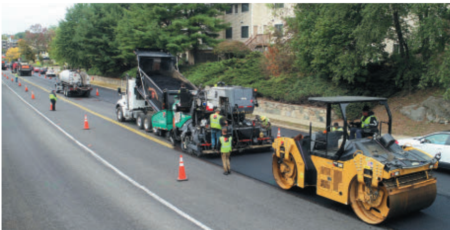
Spray paver used to efficiently place bonded wearing course in Newton, Mass
