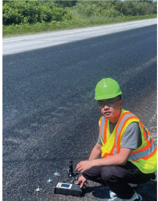
Lei Yin field-tests hot rubber asphalt chip seal project
