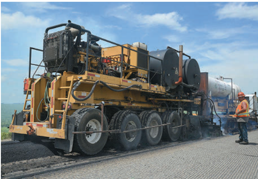
Mixer following heater is an opportunity to add rejuvenating emulsion stored in black tanks
