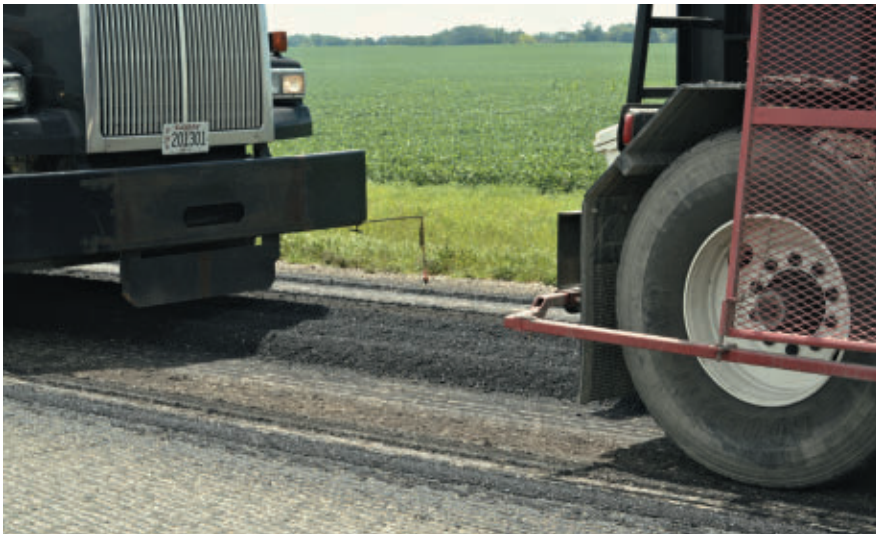
Windrow of hot recycled asphalt is maintained through the recycle train
