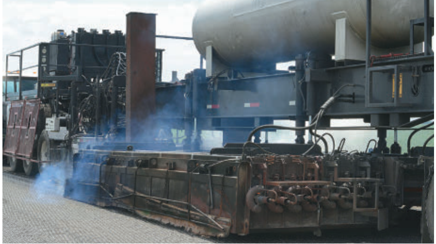
Tunnel heaters heat the underlying pavement while maintaining the temperature of the windrow
