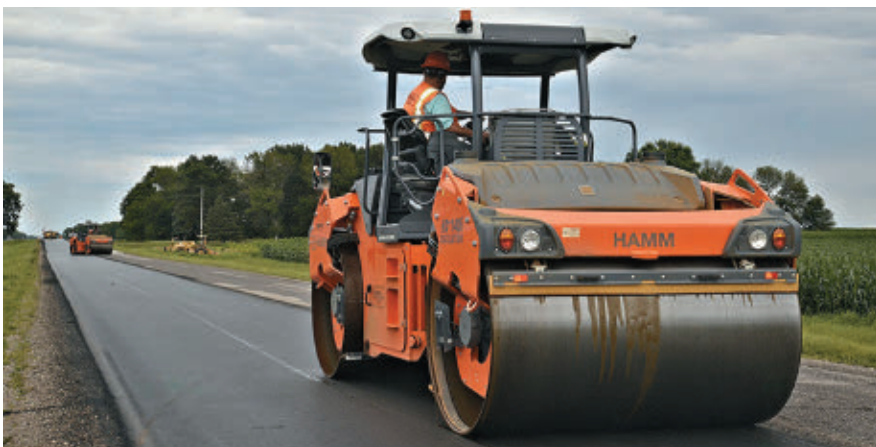
At end of recycling train, finish roller operates in static mode
