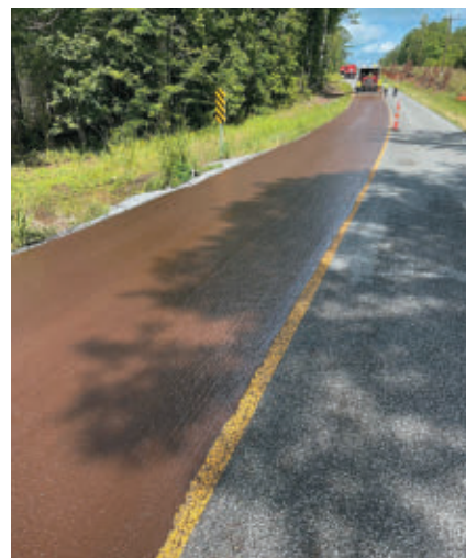
In Mississippi, contractor RJM-McQueen Contracting, Inc., Collins, Miss., places micro surfacing on top of rejuvenating scrub seal on S.R. 511 in Clarke County
