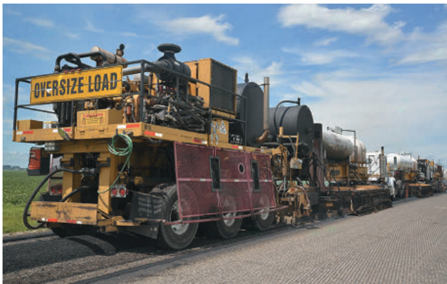
Rejuvenating emulsion added from tanks into final windrow
