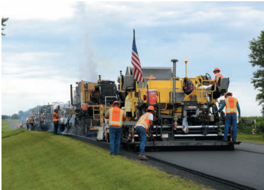
Freshly placed recycled pavement awaits breakdown compaction
