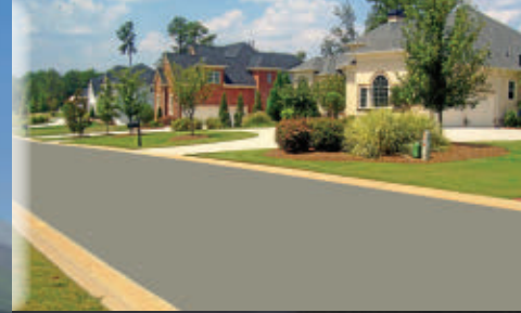
COOL PAVEMENT TECHNOLOGY
