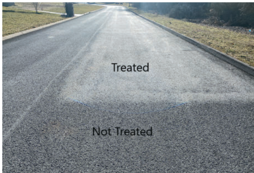
In East Tennessee in 1999 a test strip of MRT (Reclamite) on about 200 feet of pavement was placed in 1999. After more than 25 years the treated side has retained more aggregate and exhibits a denser surface matrix
