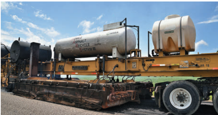
Intermediate heater continues to gently bring hot recycled mix up to optimal temperature
