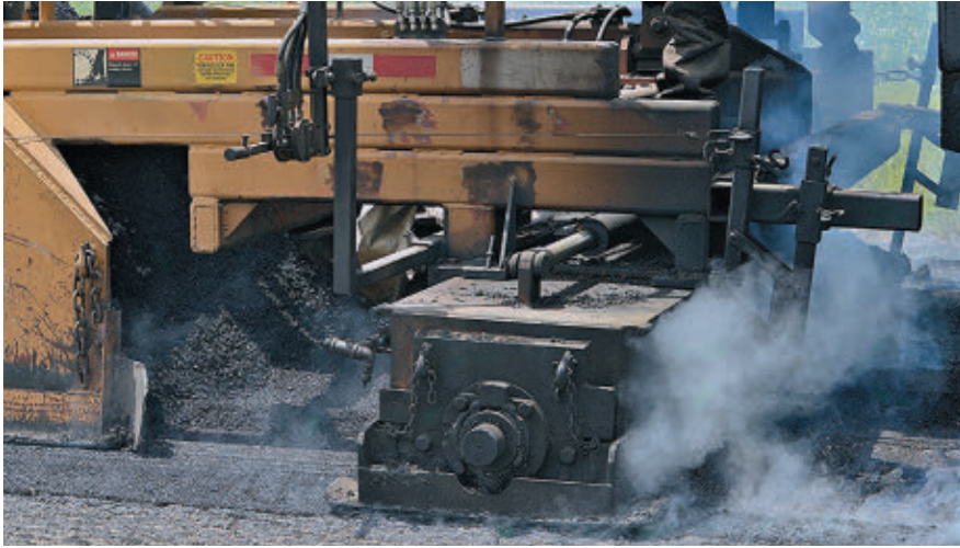
Milling drum lifts softened asphalt mix off pavement and combines with material milled earlier in train
