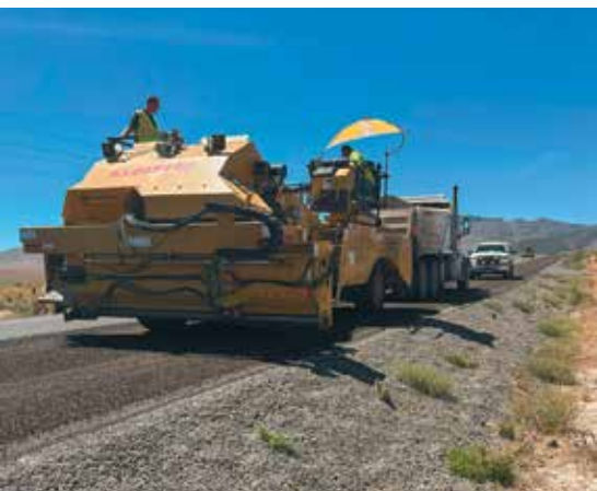
Idaho RAP chip seal under construction
