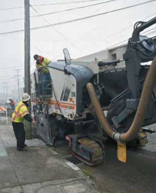
In San Francisco, overhead wires, storm sewer inlets and uneven curbs complicate asphalt milling
