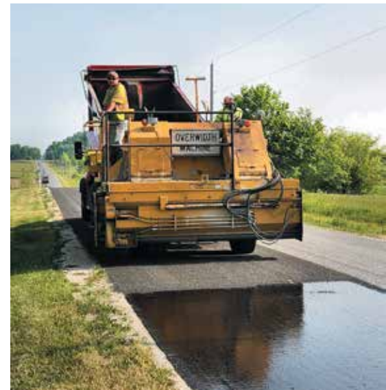
Chip seal is placed in Sheboygan County, Wis.
