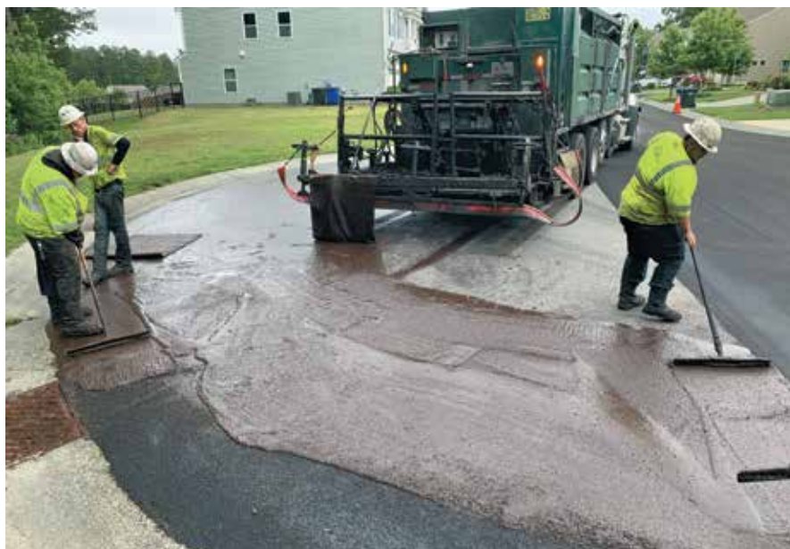
Unique features like cul-de-sacs or narrow lanes can limit equipment maneuverability, requiring specialized approaches or increased handwork
