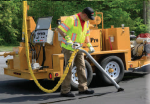
CRACK SEALING EQUIPMENT / MATERIALS
