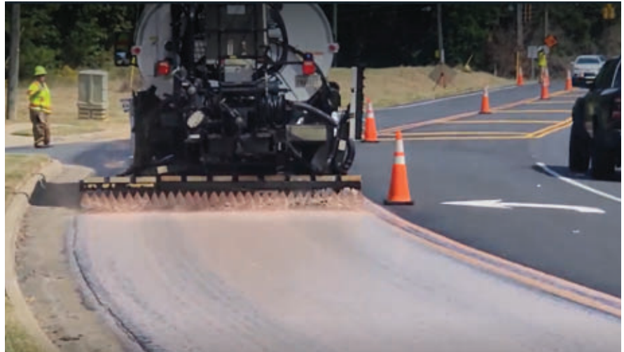
In North Carolina, application of rejuvenator with lower application rate in wheelpaths
