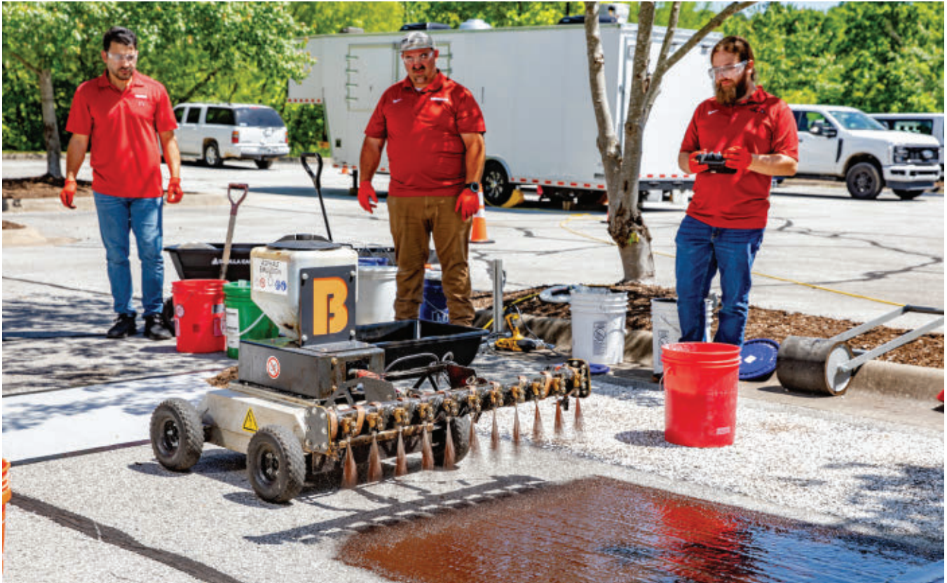
Robot mini-applicator sprays asphalt emulsion during outdoor demo
