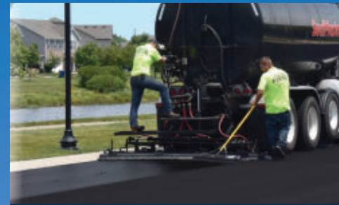
LIQUID ROAD SURFACE TREATMENT
