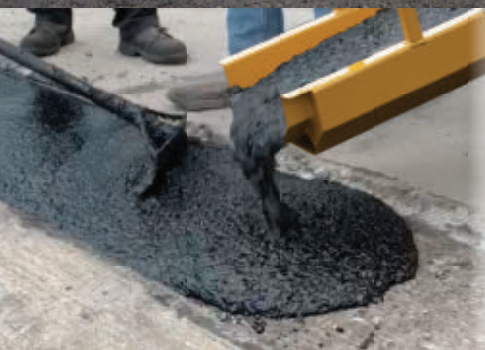
MASTIC EQUIPMENT / MATERIALS
