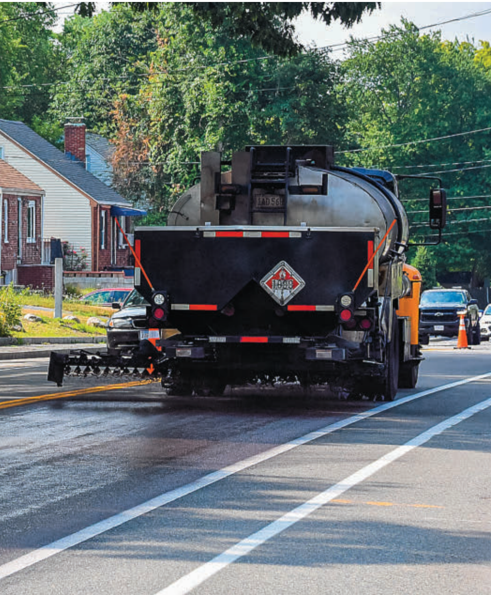
Fog seal is placed by contractor indus in Braintree, Mass
