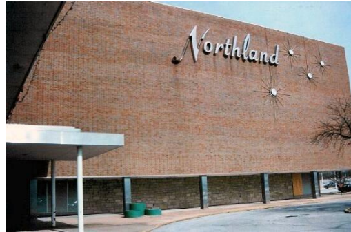
Nearby Northland Shopping Center, abandoned; in December 2004 it's being demolished.
