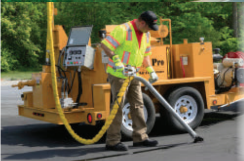
CRACK SEALING EQUIPMENT / MATERIALS
