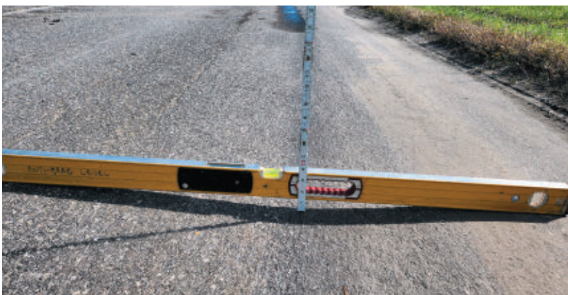
Micro surfacing fills shoulder ruts caused by horse-drawn buggies; Delaware rut during preconstruction September 2025
