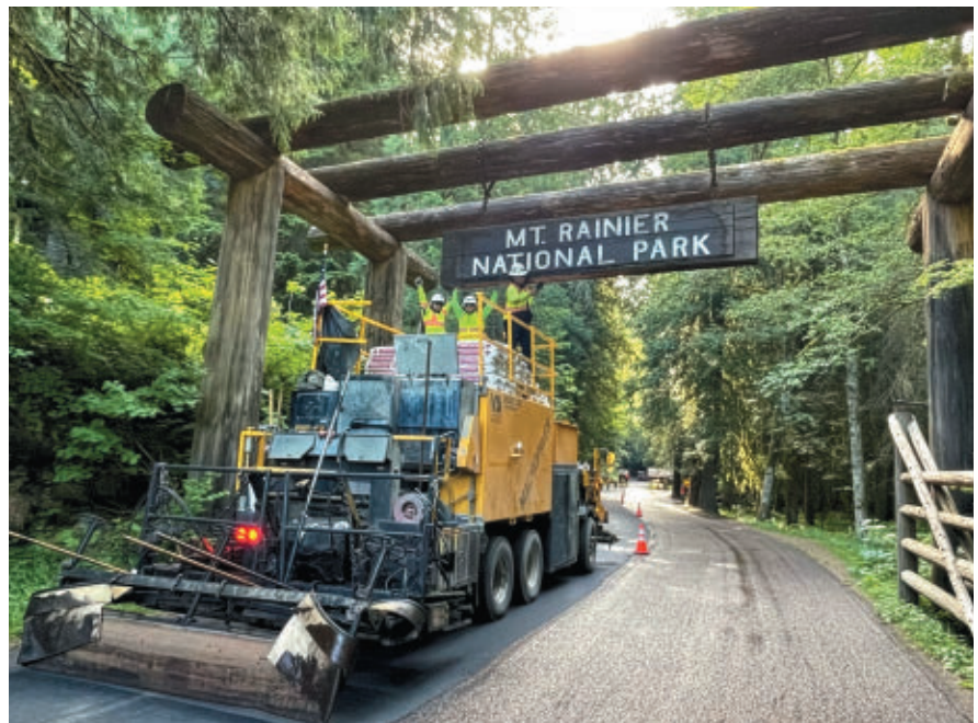
Over 650,000 sq yd of micro surfacing were placed
