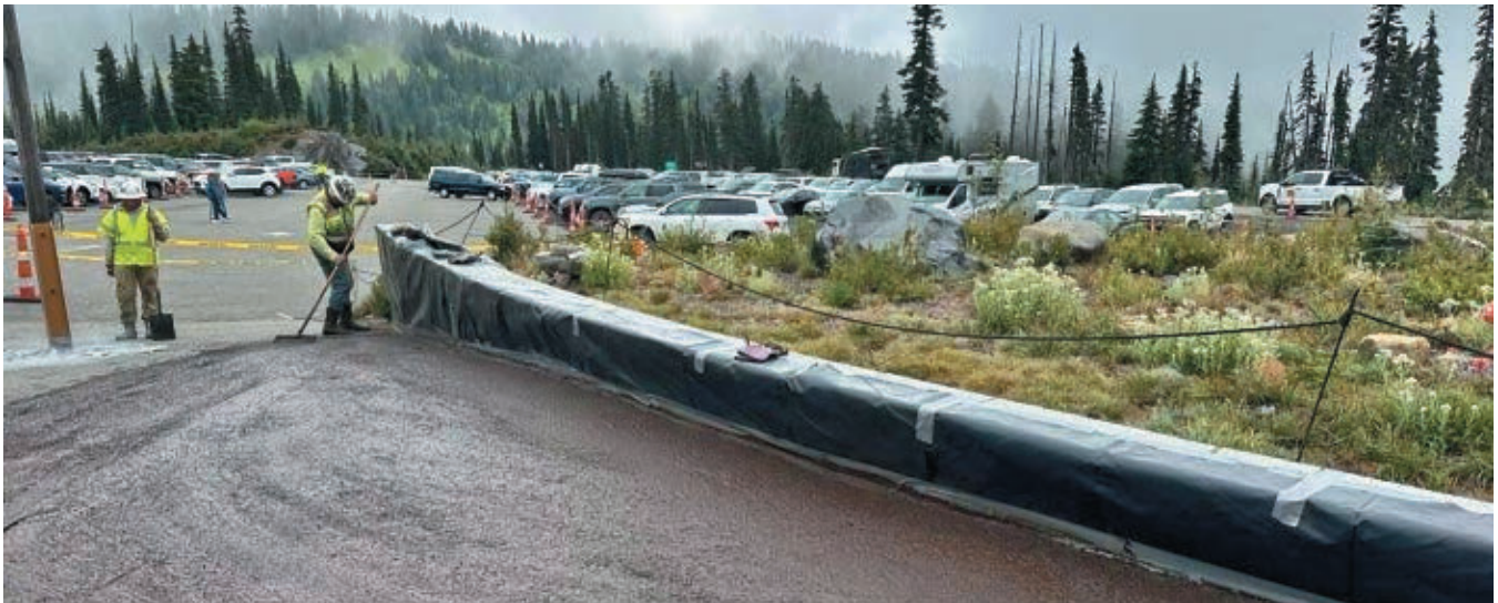
Parking areas in reserve required extensive hand work
