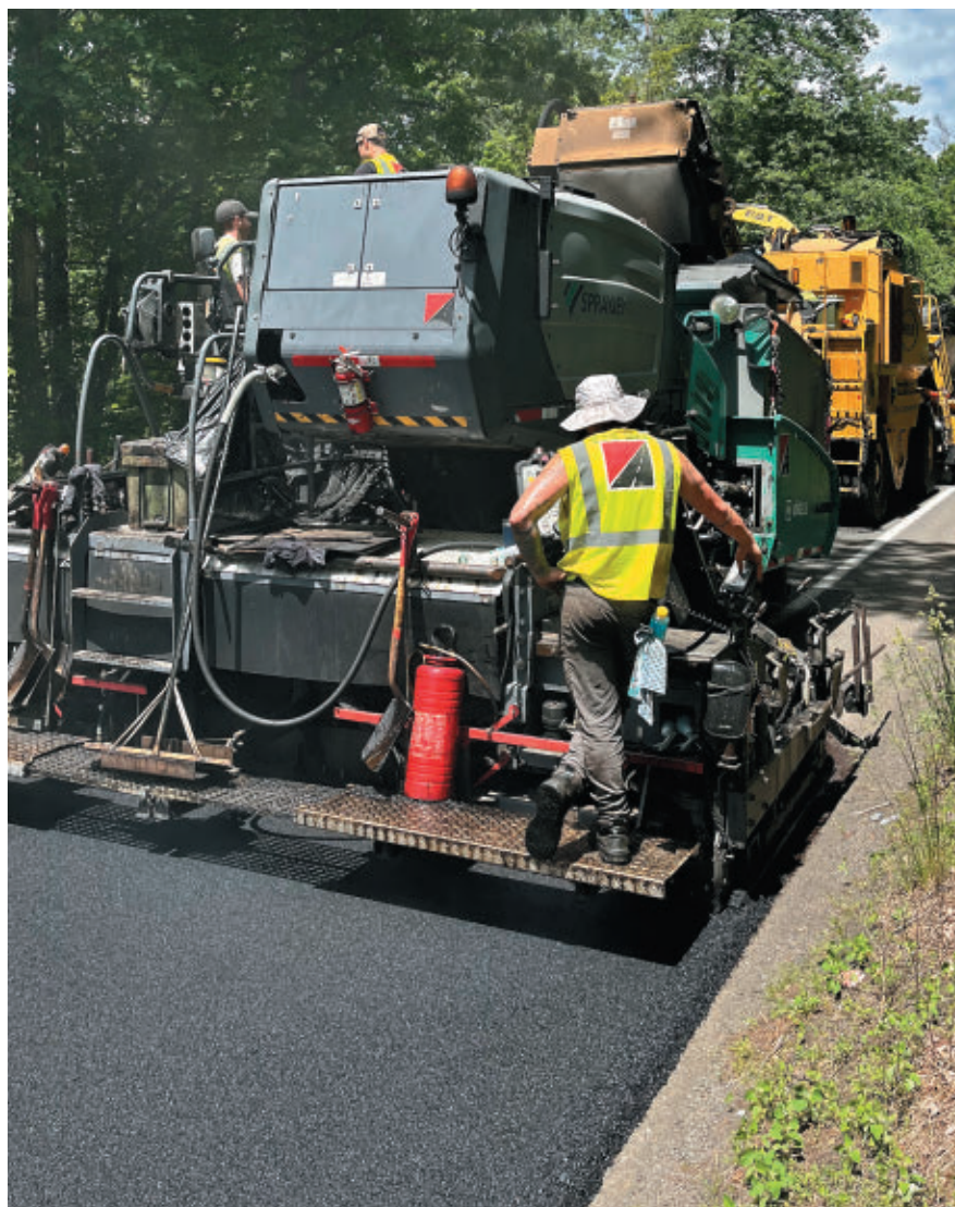
On Route 9 in Belchertown, Mass., spray paver is utilized to place a SSC 9.5 polymer mix in one pass
