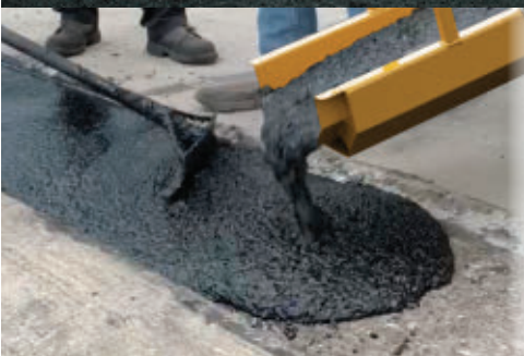
MASTIC EQUIPMENT / MATERIALS
