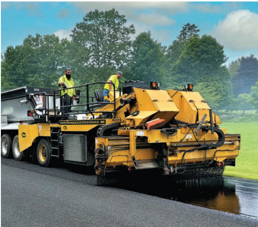
Rubber chip seal placed on Mass Route 32 in Hardwick, Mass.
