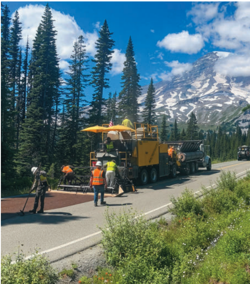
Macropaver at work approaching ramparts of Rainier
