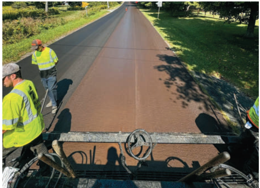
Micro surfacing is placed on Mass Route 41 in Alford, Mass.
