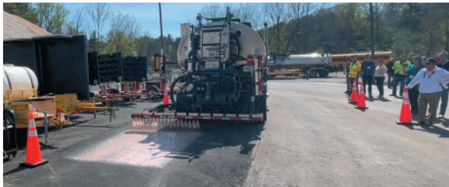
Rejuvenating asphalt emulsion (pink) is placed by FP 2 supporter Pavement Technology Inc. at outdoor SEPPP demo
