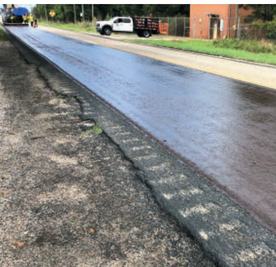
Micro Surface applied to the Scrub Seal on SR 109
