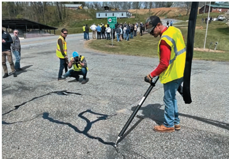
At SEPPP meet, Crafco representative demonstrates crack sealing best practice
