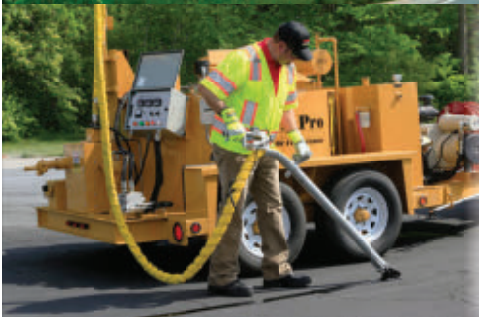
CRACK SEALING EQUIPMENT / MATERIALS
